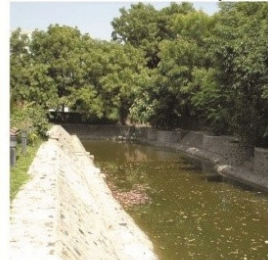
Rain water harvesting
