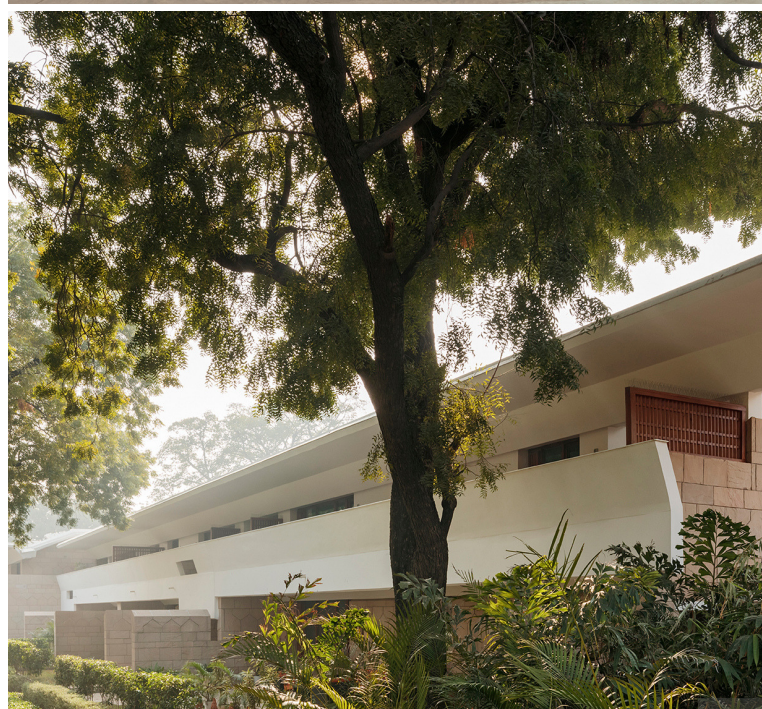
Natural sandstone facade with white plastered bricks.
