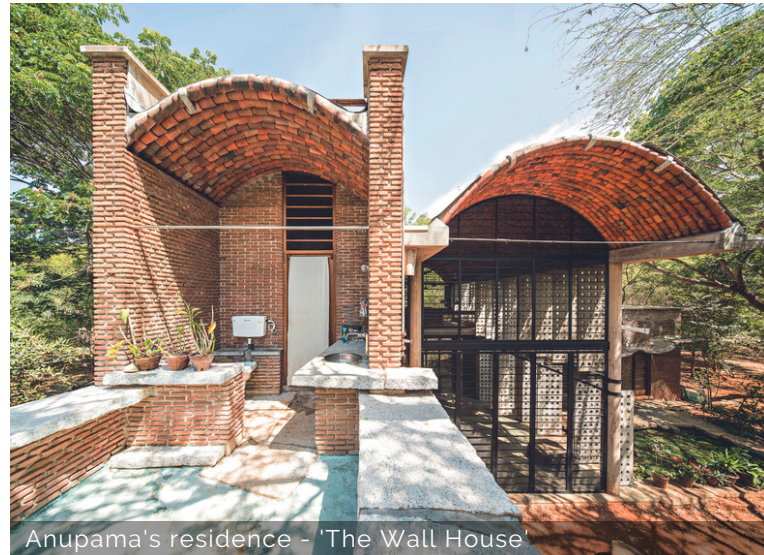
The domes are sustainable in all aspects.
