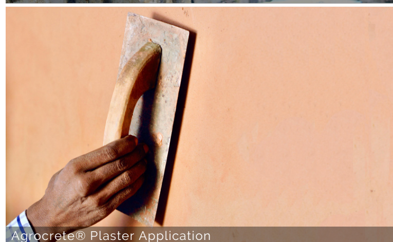
Agrocrete® wall under construction
