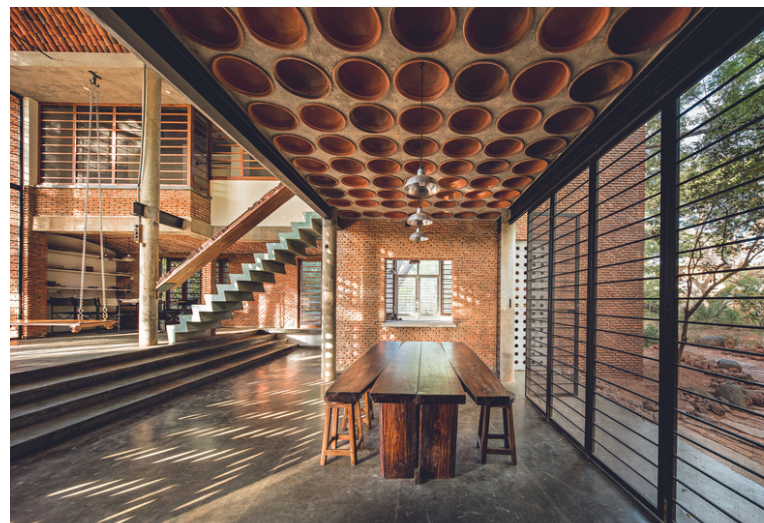
Catenary vaulted roof is used for climatic insulation.
